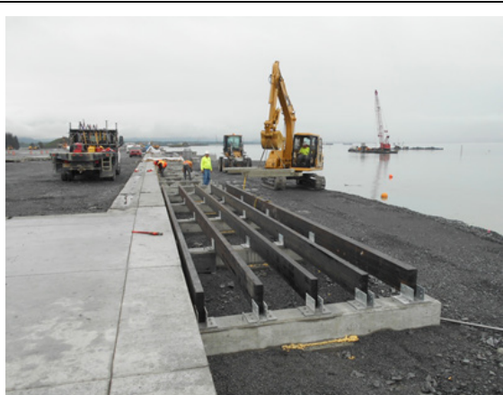
Placing glulam beams in saddle brackets
