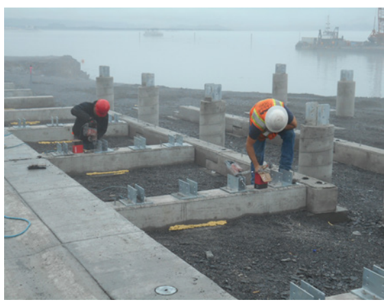
Installing saddle brackets to boardwalk sleepers
