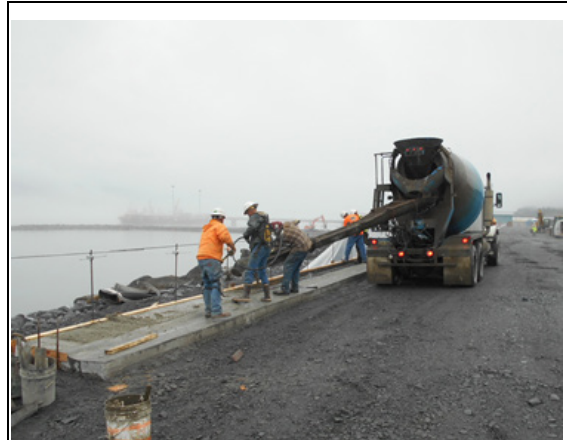
Placing concrete for sidewalk along boardwalk
