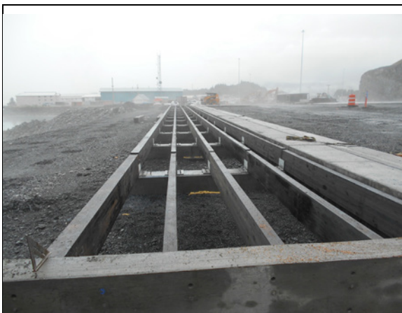
Beams ready for placing timber decking
