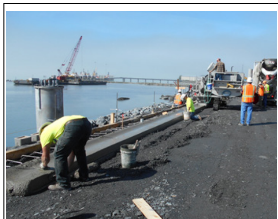
Hand finishing concrete curb placed by machine
