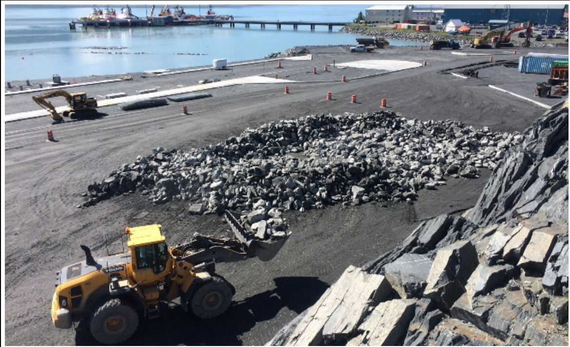
Western Marine sorting and loading rock for breakwater
