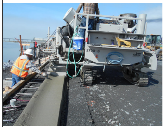
Machine places concrete curb without forms
