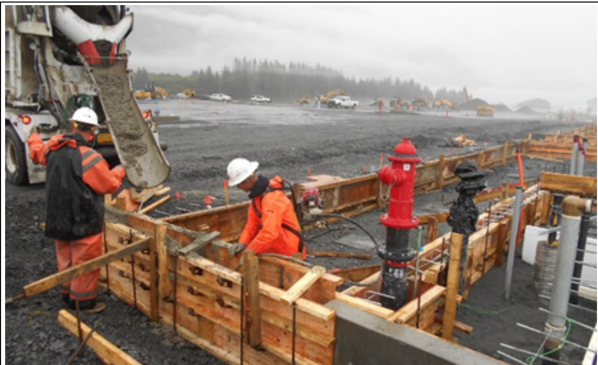
Placing concrete in stemwall forms near utility pad area
